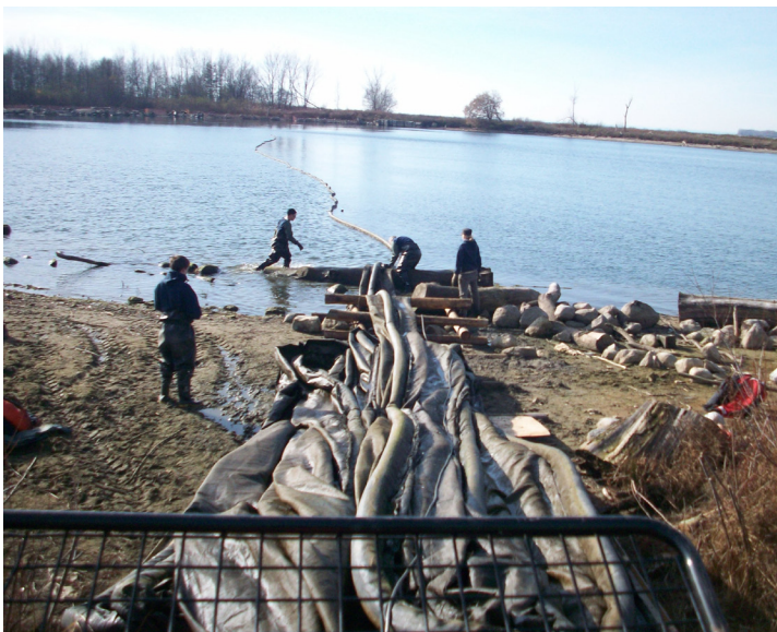
Silt curtain removal in a Tommy Thompson Park embayment
